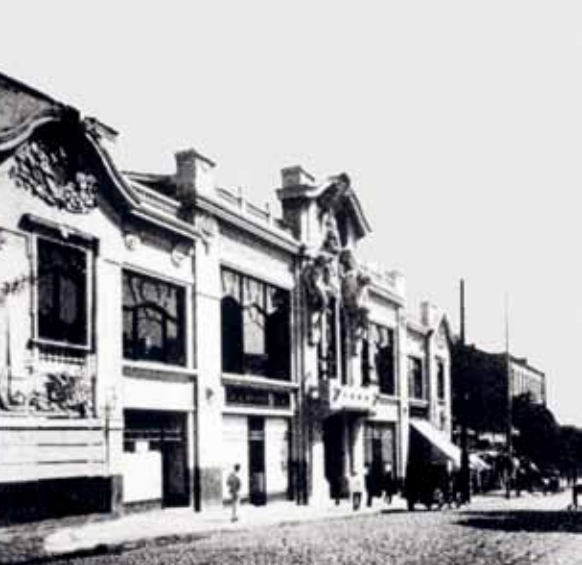
Central Bank in Georgia was first established in 1919
